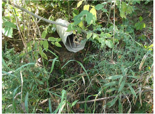
CV007TMM Bearing: OUTLET Date: 09/11/2019
