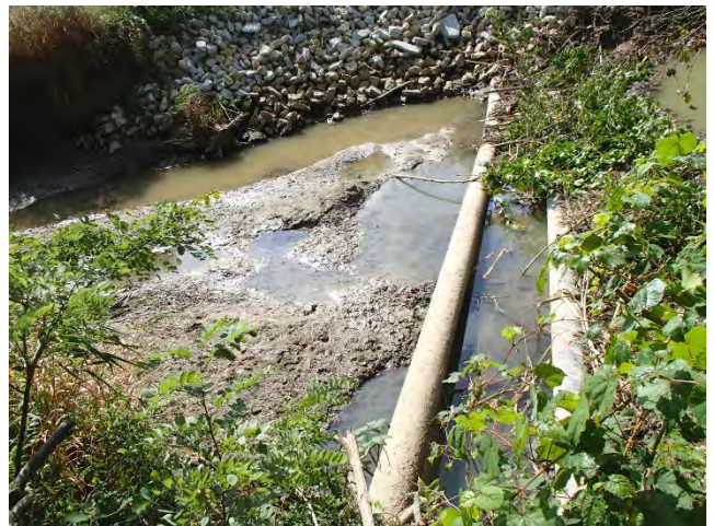
ST003TMM Bearing: WEST Date: 09/11/2019
