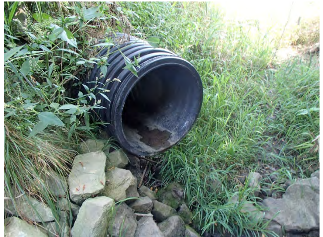
CV005TMM Bearing: OUTLET Date: 09/11/2019
