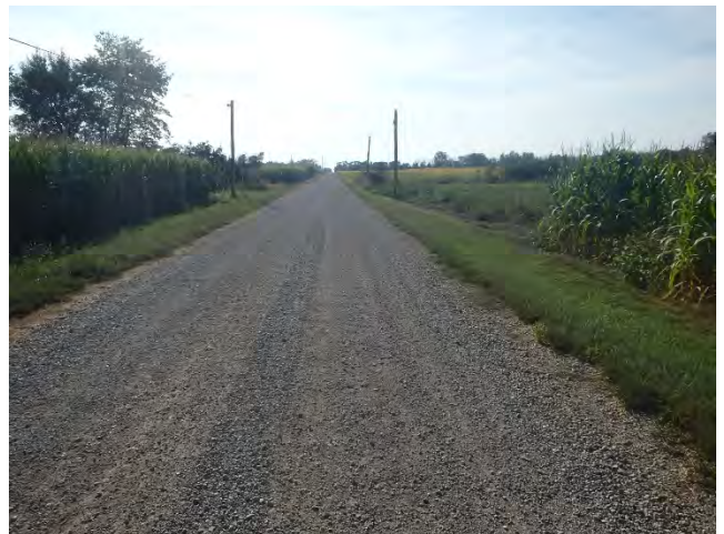
RU010TMM Bearing: EAST Date: 09/10/2019
