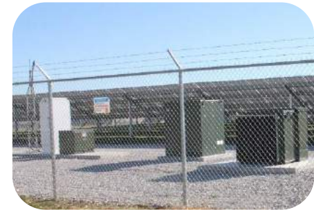
Site secured with a 7' chain link fence with 1' barbed wire
