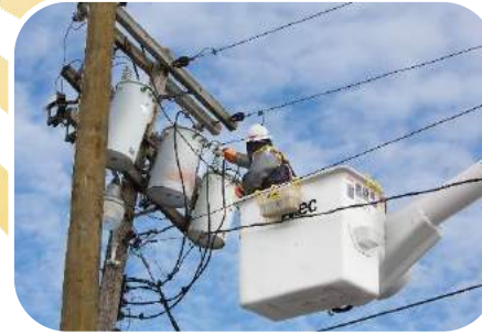
Interconnection with Members' electric distribution system
